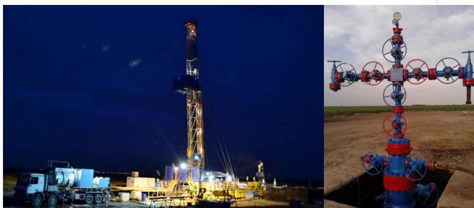
Figure 3 - Jimbolia-100 Well - wellsite (night view), Xmas tree
