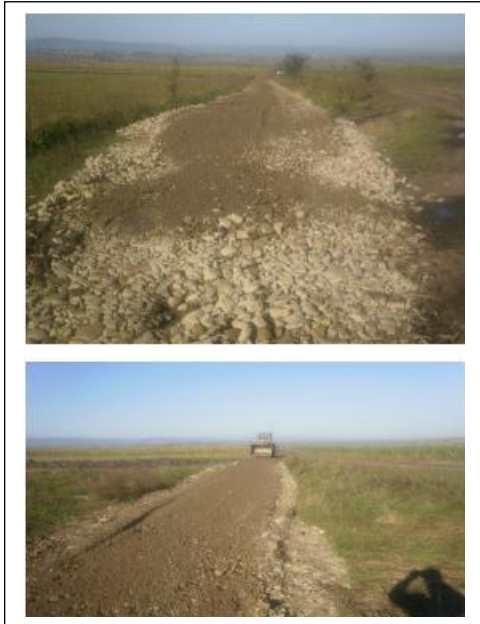
Musenita-1 Well: Road construction
